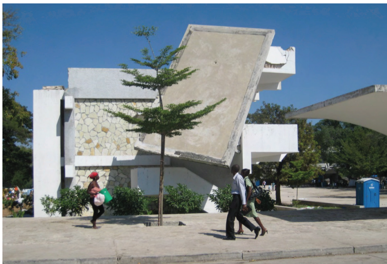
Figure 13 - Hanging debris: A simple example of an ongoing building hazard (Photo credit EES)
