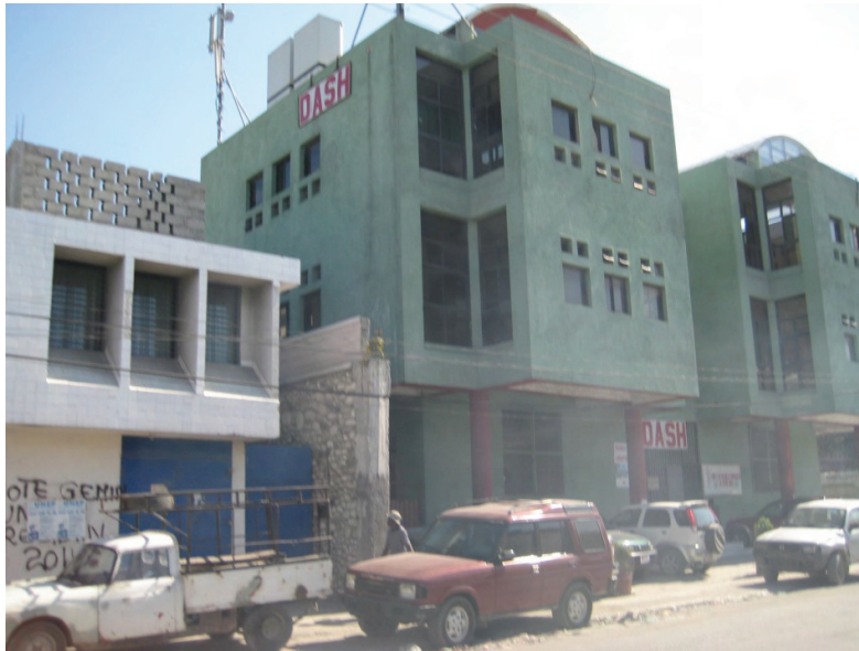
Figure 9 – DASH Delmas 48 Hospital – Sound and undamaged but evacuated (Photo credit EES)
